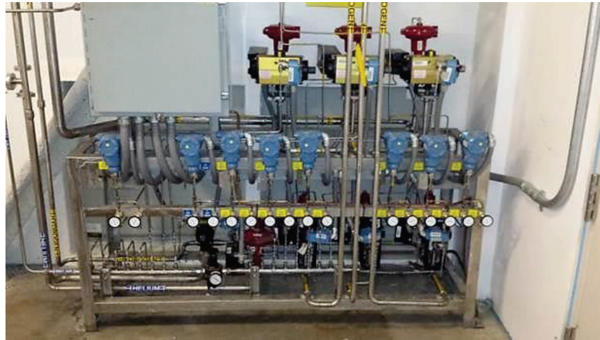
Fig. 4.24. FTS hydrogen gas management system.
