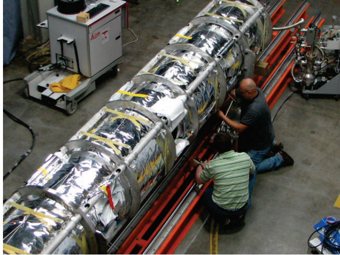
Fig. 3.26. Cryomodule cold mass assembly
