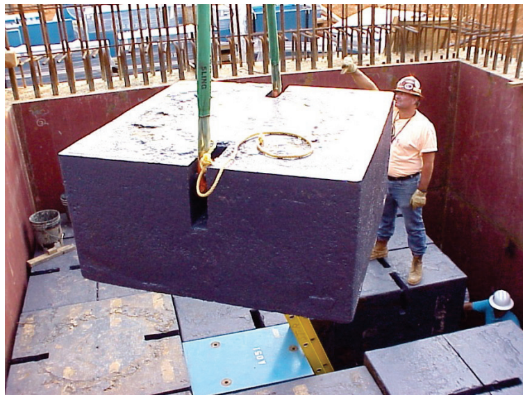
Fig. 4.40. Recycled steel block placement in FTS beam dump.
