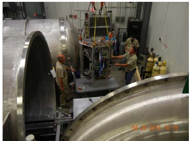
Figure 10: Lifting the detector for installation
