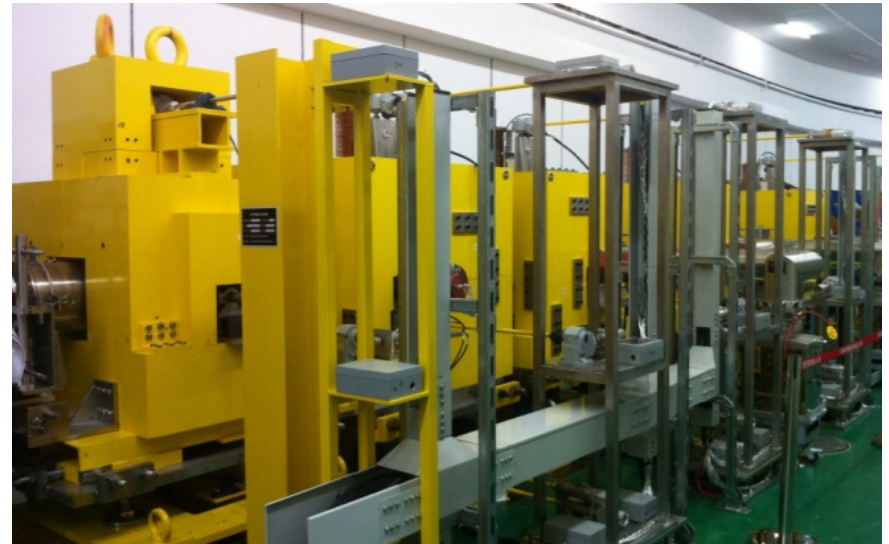
Installed collimators in RCS tunnel
