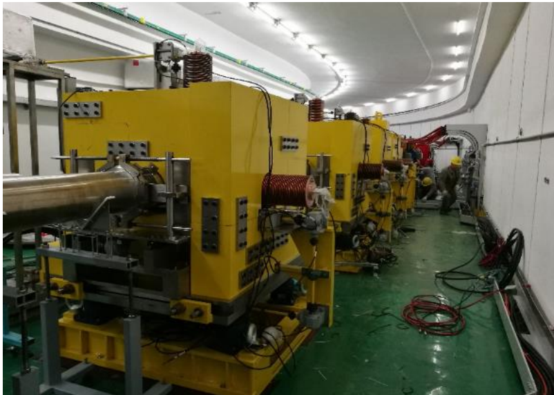
RCS Collimator Installation
