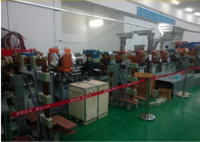
RCS Ring Injection Area Installation
