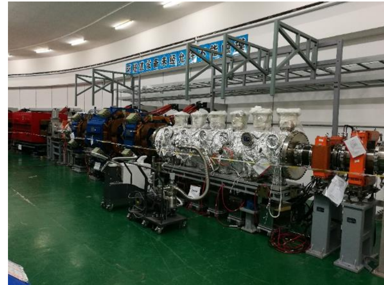
RCS Extraction Area Installation
