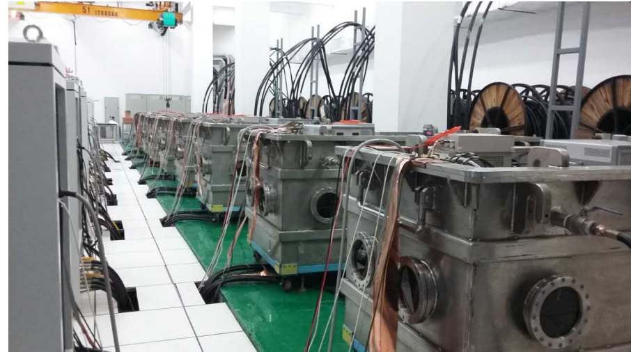
Mass production of RCS kicker power supplies
