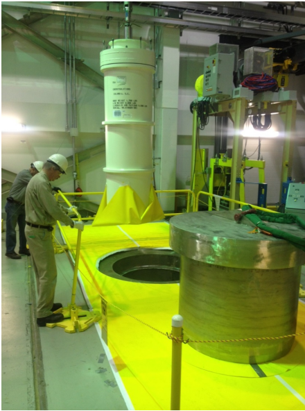
Figure 2. High Bay view of inner liner and open top loading port. Note the top loading port shielding plug in the foreground.
