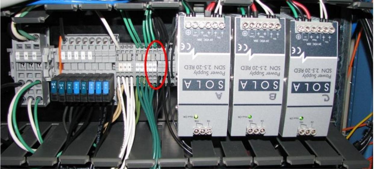
**Photograph 3.** Actual Photograph of Improperly Installed Jumper Causing PPS Failure. (Note the improperly installed jumper circled in red.)
