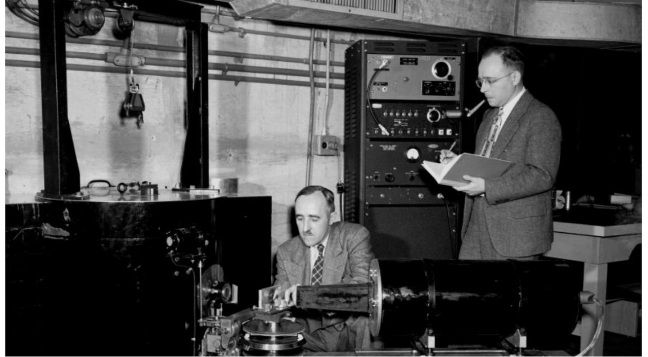
Neutron scattering pioneers, Ernest Wollan (left) and Clifford Shull\* work with the first instrument exclusively for neutron scattering, a double-crystal neutron spectrometer, **at the ORNL X-10 Graphite Reactor in 1949.** (\*C.G. Shull was a co-winner of the 1994 Nobel Prize for the development of the neutron scattering technique.)
