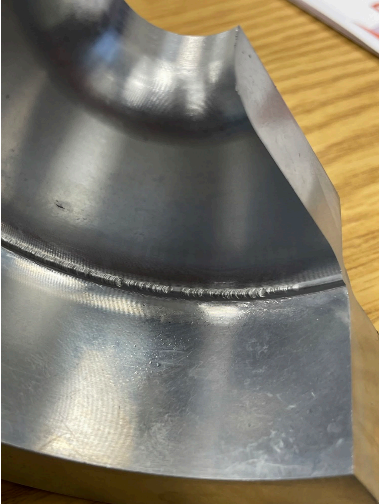
Over penetration of vacuum vessel weld backer resulting in melting of backer.
