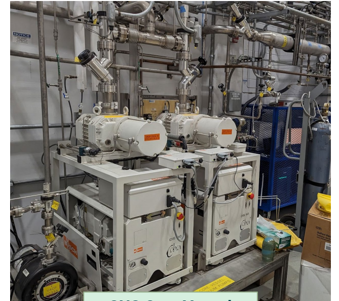
SNS Core Vessel Vacuum Pump Station
