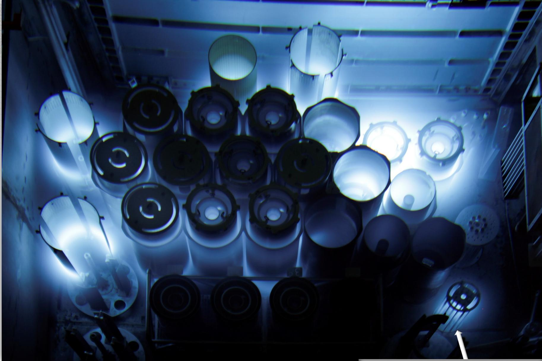
The most recently used fuel element is glowing most brightly
